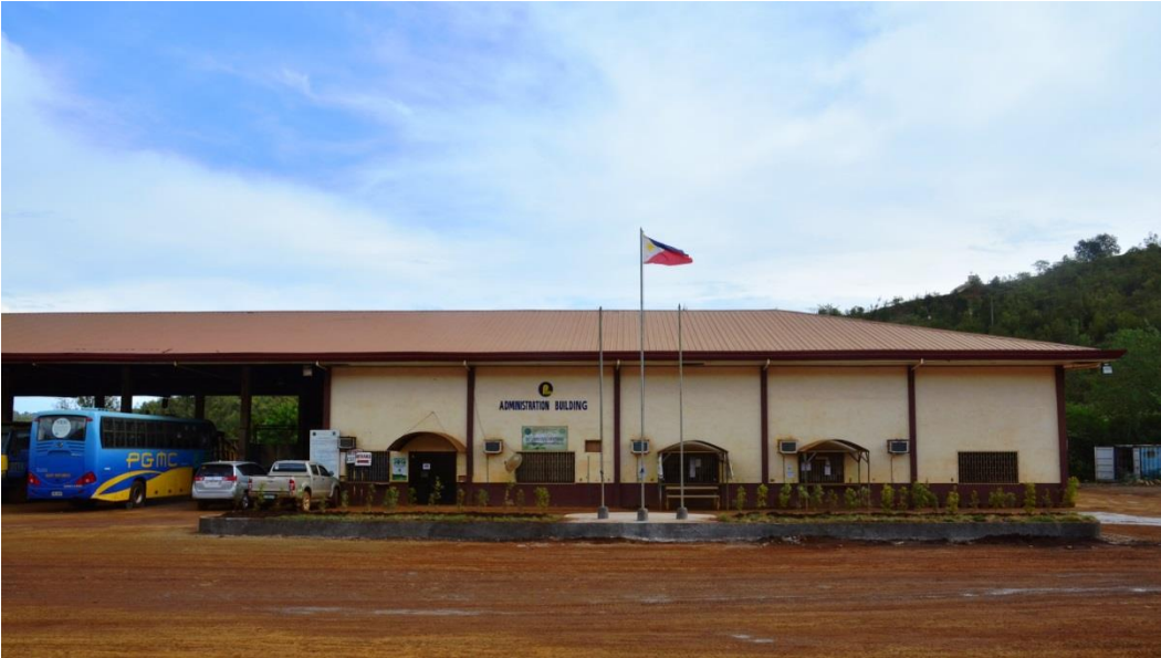
Figure 122. Existing Administration Office
