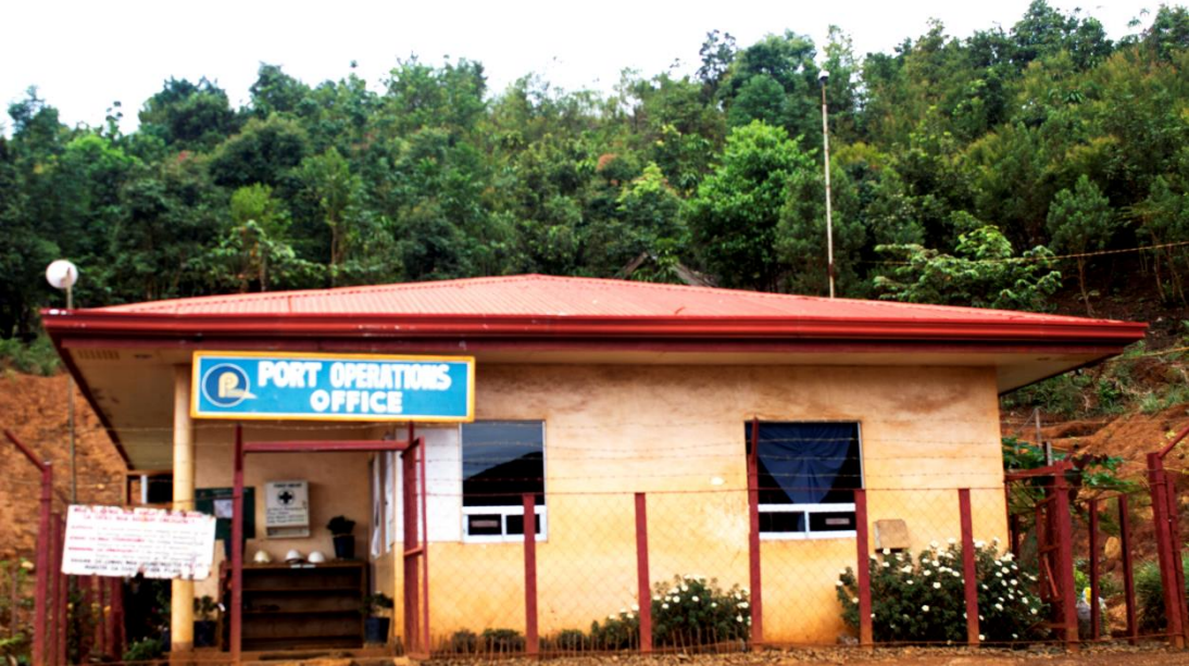
Figure 131. Port Operations Office
