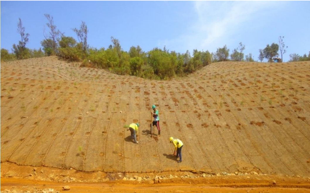
Figure 143. Coco Nets for slope stabilization
