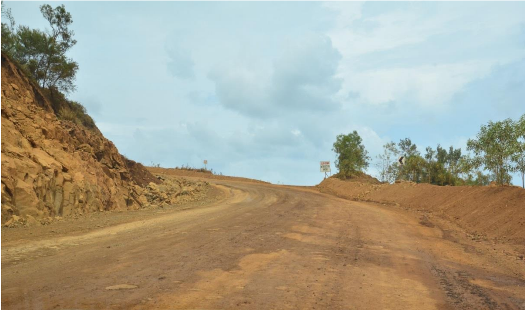
Figure 134. Existing Mine Roads
