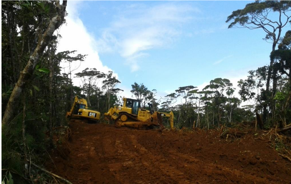
Figure 114. Removal of vegetation thru clearing and grubbing
