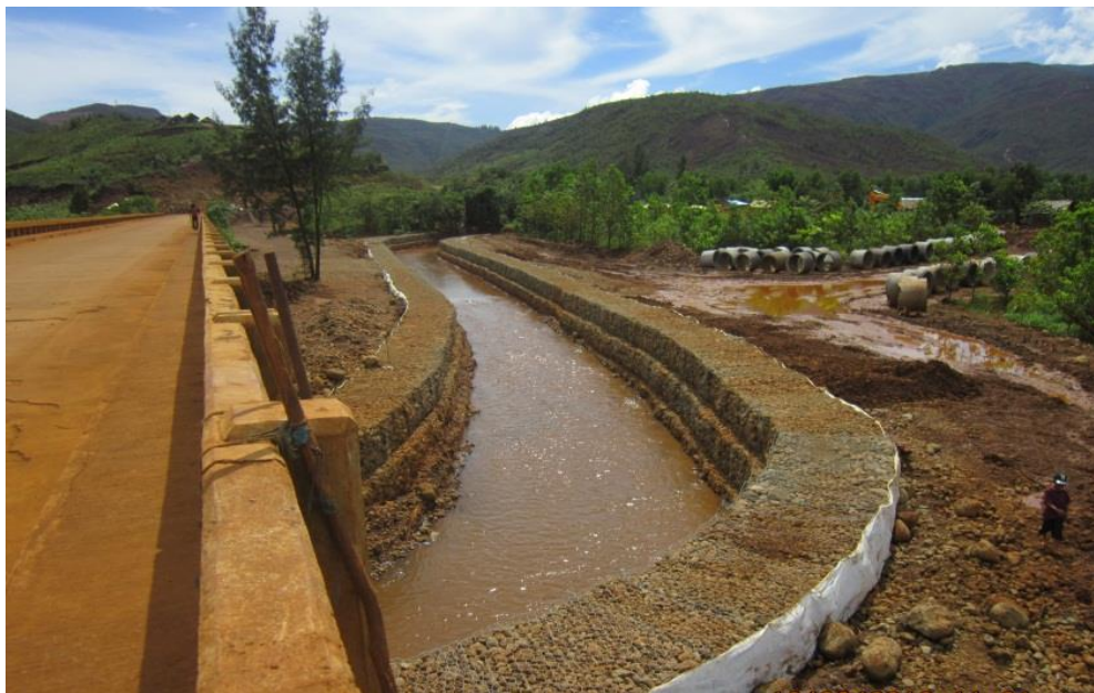
Figure 141. Gabion structures as river bank protection
