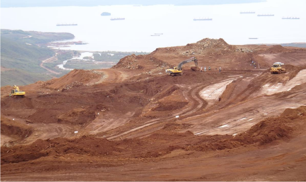
Figure 135. Block 6 at CAGA2 pit
