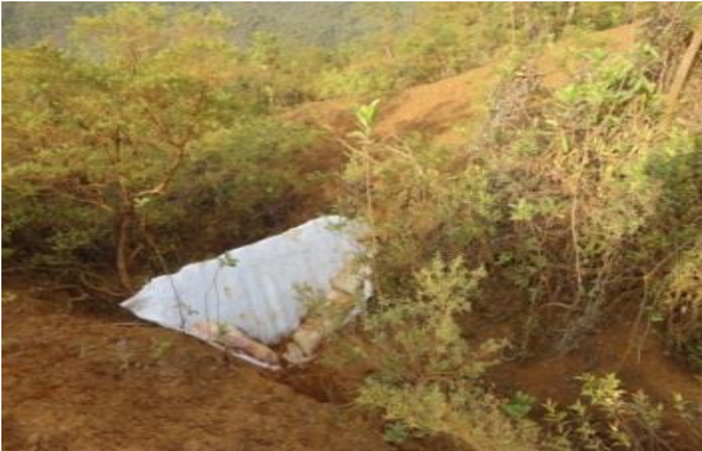
Figure 142. Silt traps and fences with geotextile
