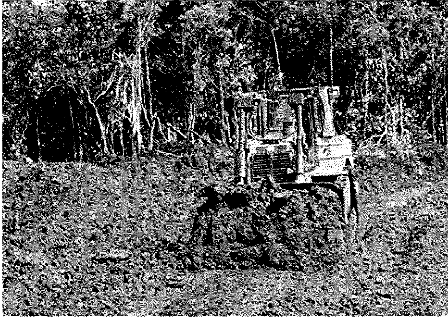
Figure 126. Removal of vegetation thru clearing and grubbing
