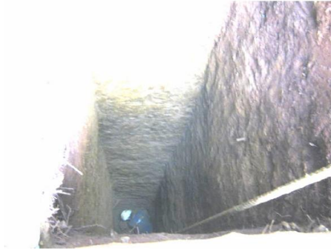
Figure-24. Test Pitting Excavation (Source: TMM)
