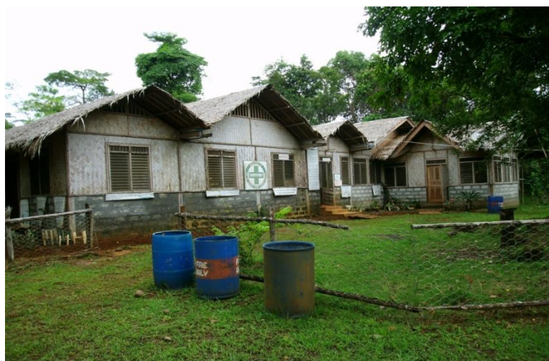
Figure-54. Geotechnical Investigation Site
